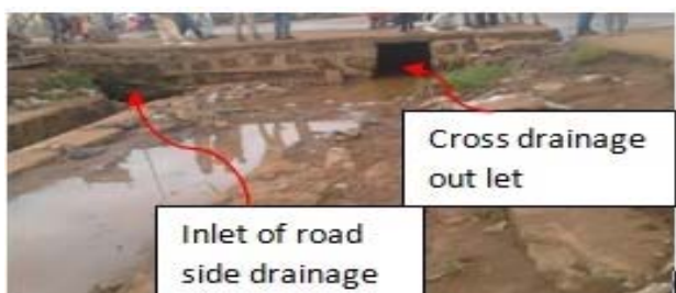
Figure 7: Damaged road and drainage.
