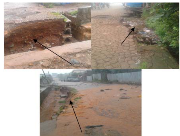
Figure 7: Damaged road and drainage.
