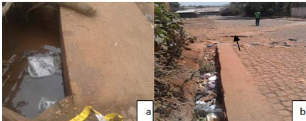
Figure 4: Cross drainage filled by sedimentation and solid wastes; (a) on the route bus station gate to Maedot (b) Back of US College.
