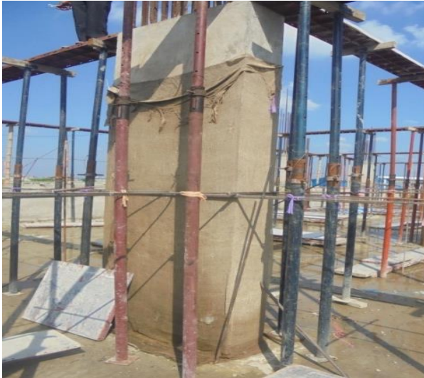
Figure.1Curing of Concrete
