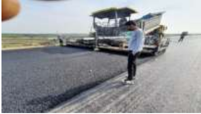
Fig.1 Survey Under construction
