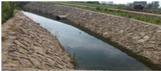
Fig 1. Plate (1) Part of the lined canal.
